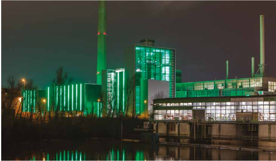
Powerstation Fortuna, operated by Netzgesellschaft Düsseldorf
